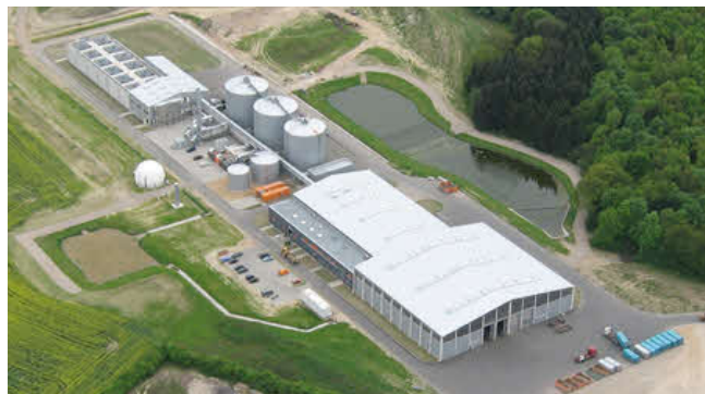
MBT Treatment Facility in Belfast but not in Norfolk
