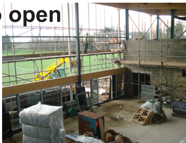
Work progressing on the main hall
